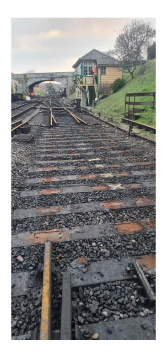
After P'Way has been along and taken up the track and then replaced it, there's more work for the Signal and Telegraph department (S &T) to ensure the points are adjusted and the track circuiting reinstated.
