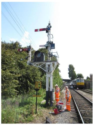
And checking the operation of the calling-on signal on the inner home signal post. John Blyth is on the phone to the signalman, while Paul Smith, all the way from Spain to help out, pauses from painting the shunt signal apparatus.
