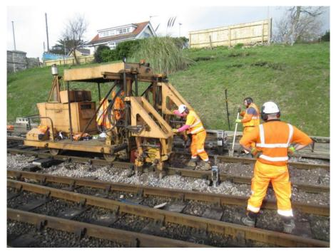
Here, one of the workers directs the tamper operator to avoid damaging any equipment between the rails and sleepers.
