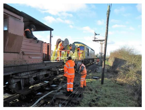
On 23rd January, Signal and Telegraph volunteers roll out new signalling cables to replace those slung from the less-than-upright poles, which have seen better days.
