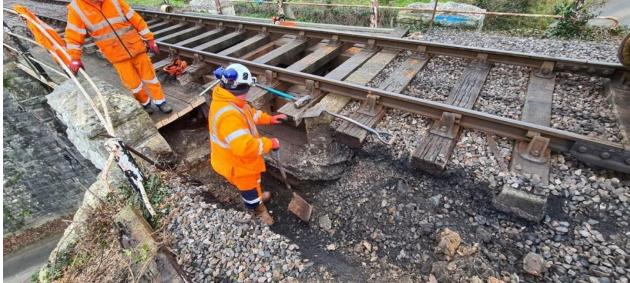
Also on  $6^{th}$  January, they've been exposing the bridge beams at New Barn, above, prior to a bridge inspection on  $7^{th}$  January below.
