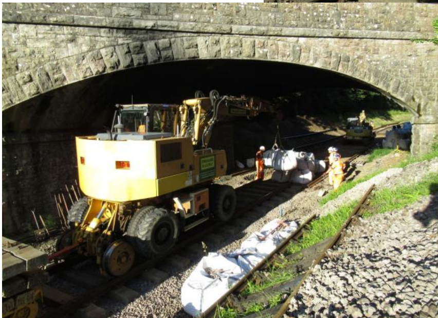
Richard Fry in Little Sis levels the new ballast. Must have laser eyesight for this job!
