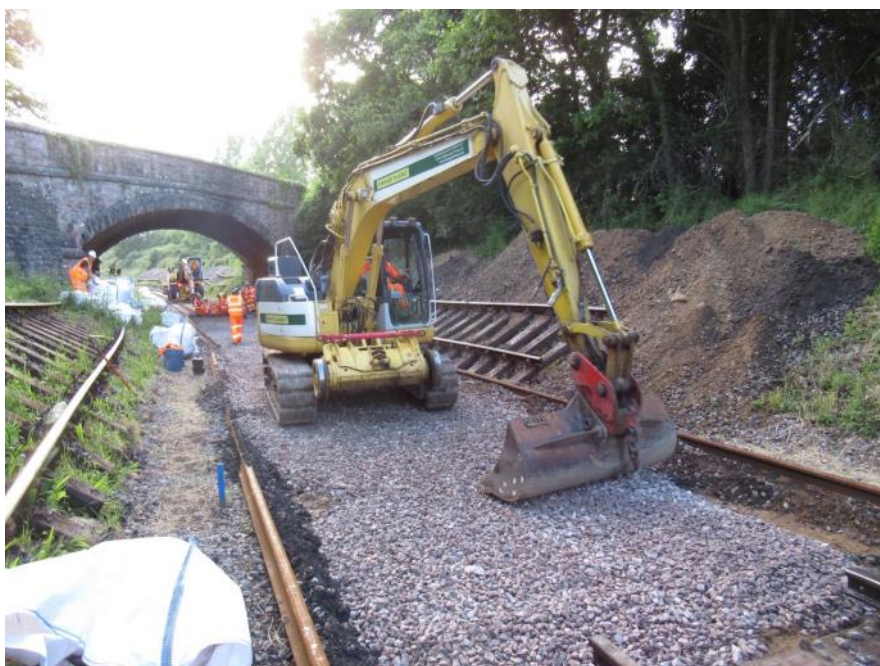
Richard Fry in Little Sis levels the new ballast. Must have laser eyesight for this job!
