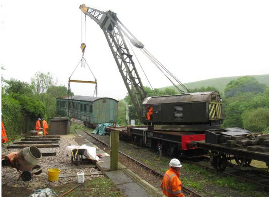
At Corfe, the coach is lifted into position onto a prepared bed of timbers.
