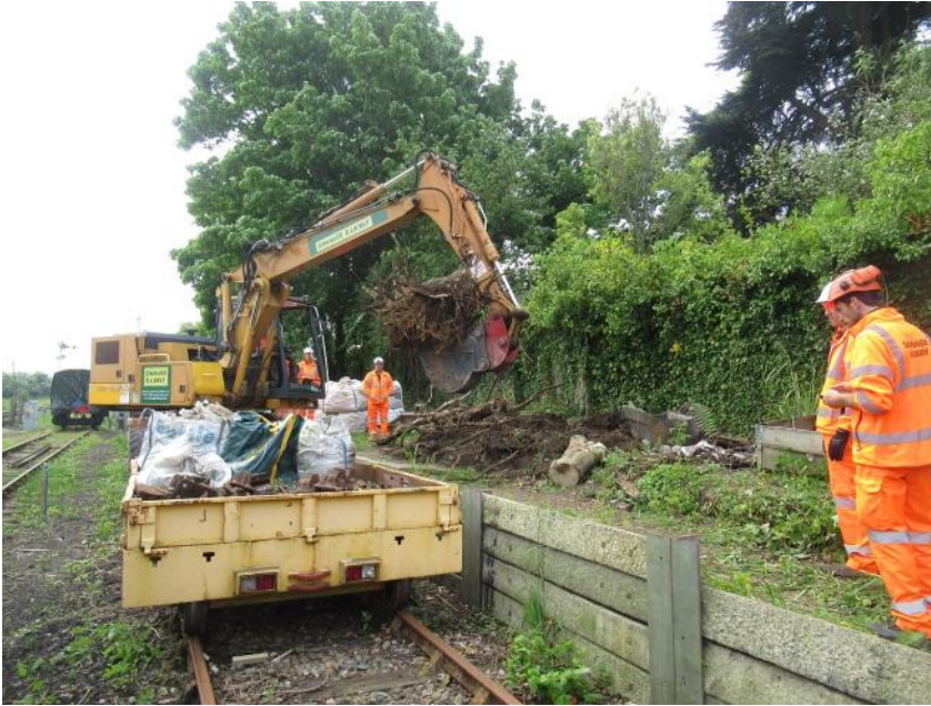
On 22nd May, the sidings at Corfe have been emptied and our P'Way team is setting about preparing a site for the re-location of the wooden coach body recently removed from Swanage (see issue 33).
