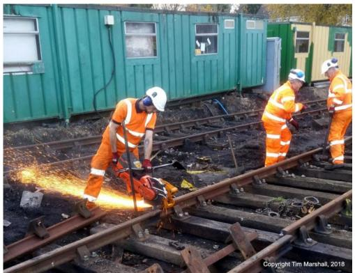
On 14th November, the track is being re-laid, and Tim's picture shows Tyler Herrington trimming a rail to fit.
