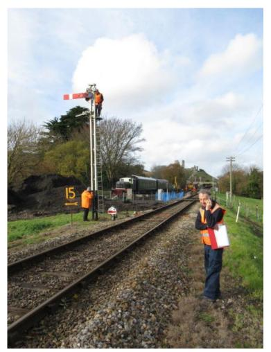
Further on, an attempt is made to check the operation of the Up Home signal. This has to be a limited inspection as it is not possible to operate the signal with the track ahead occupied by the works train.
