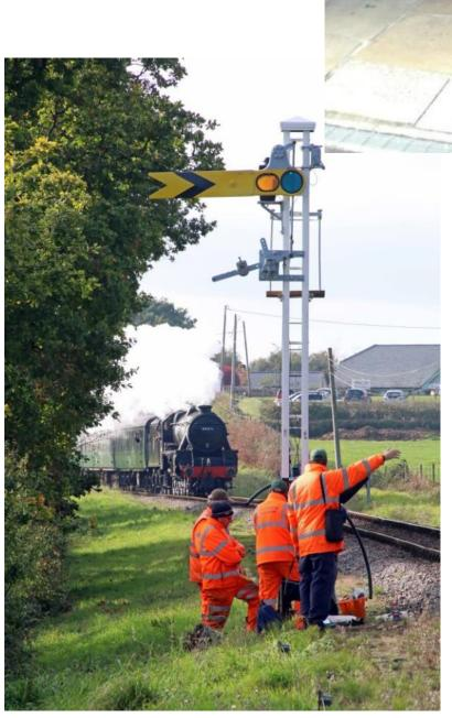
Down the line on 25th October, the Black Five has just left Harmans Cross station towards Swanage and is about to pass the Signal and Telegraph technicians, who have just commissioned the re-located Harmans Cross Up Distant signal.
